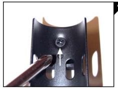
Using a phillips head screw driver, install the provided #6 x 3/8" screw at the rear of the heatshield as seen in Figure 4. Make sure the ghost ring sight is centered before the screw is tiahtened.
